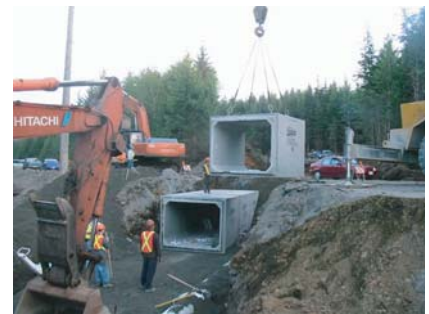
Placement of culvert below Hwy 19 for ship loadout conveyor
