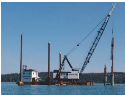
Pile driving at Orca Quarry underway
